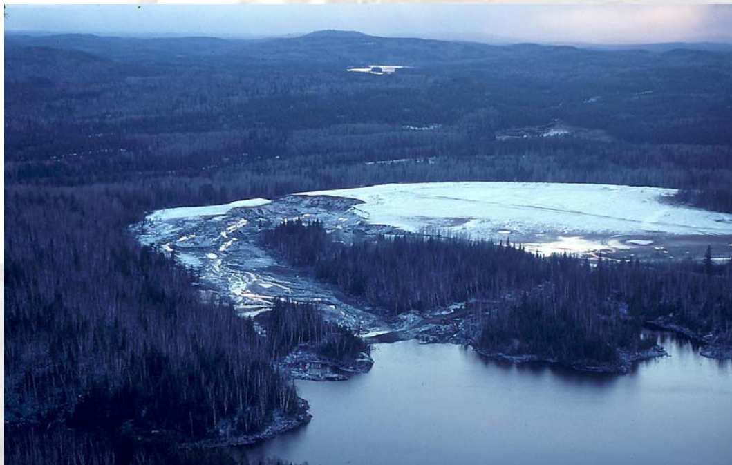
Photo 9: Run-out of poorly managed mine tailings.
