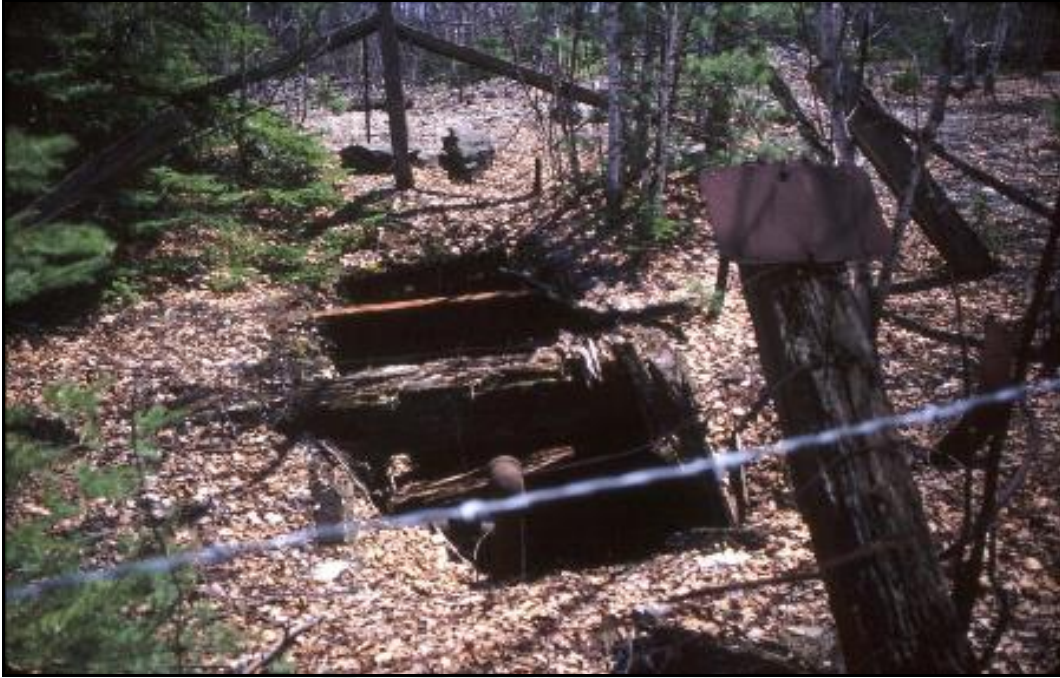
Photo 2: Abandoned, unprotected mine shaft works.
