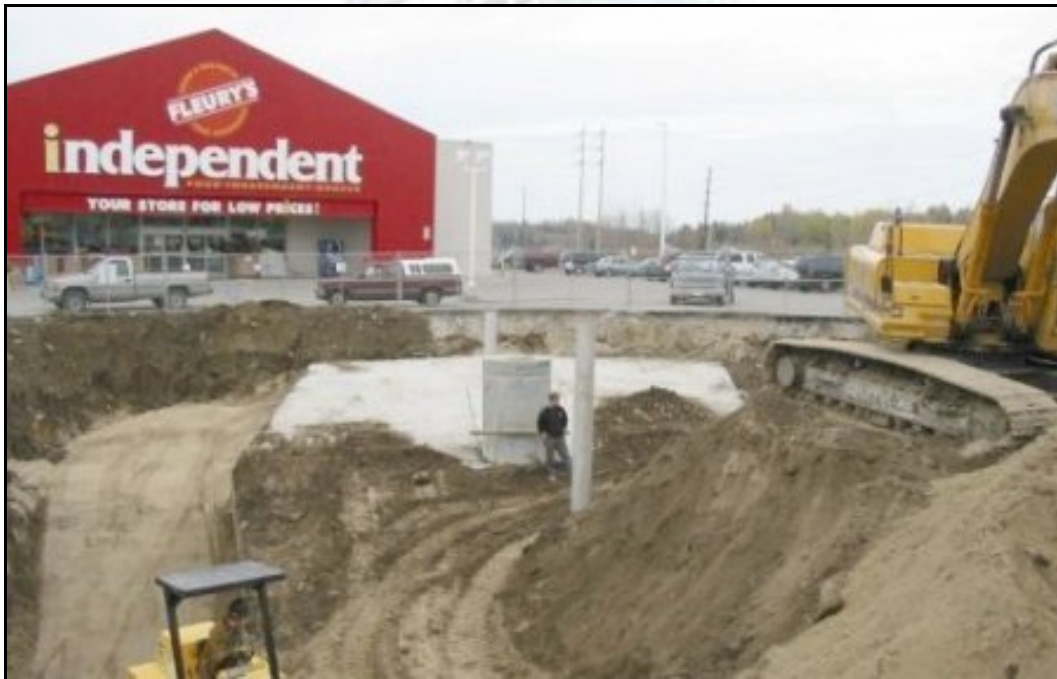
Photo 6: Construction of cap over unsafe underground workings (source MNDMF).
