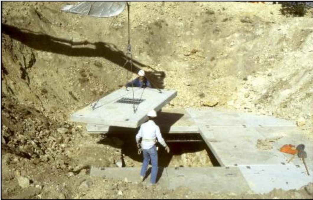
Photo 3: Placing a removable shaft cap.
